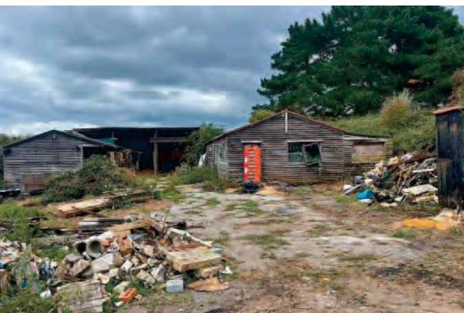
Clearance work at Marina Farm by J E Green Ltd
